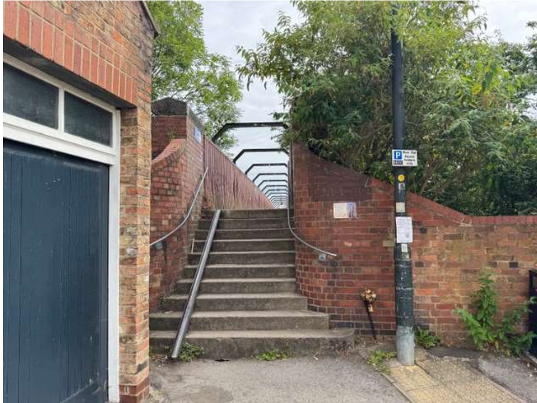
Existing access from Wilton Rise
