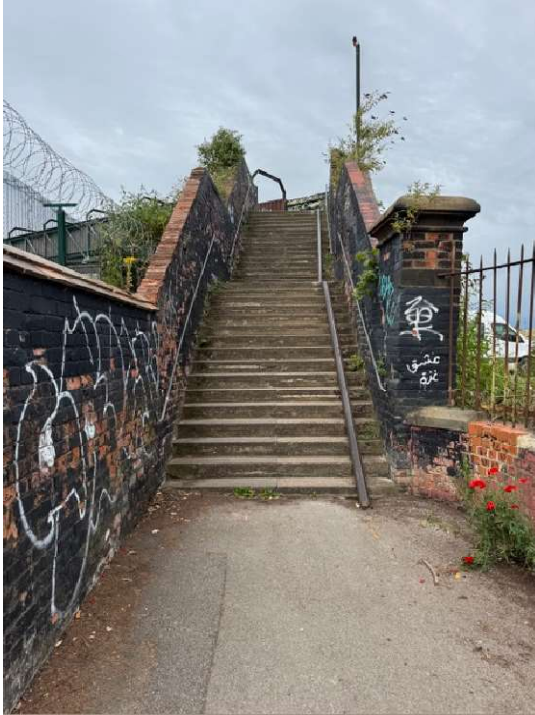
Existing access from Cinder Lane
